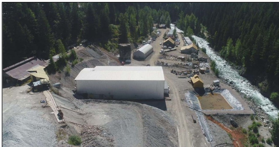
Bralorne Facilities Bralorne, BC, Canada
