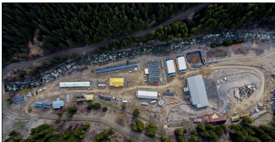
Bralorne Facilities Bralorne, BC, Canada
